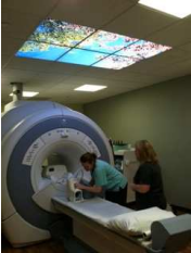
26ft L x 19ft W MRI room 3T magnet 8 LED 1x4 fixtures 6 LED 1x4 Sky Mural
